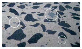
Holes filled when grinding with 120 grit metal-bonded diamonds and GM  $3000^{\text{TM}}$ .
